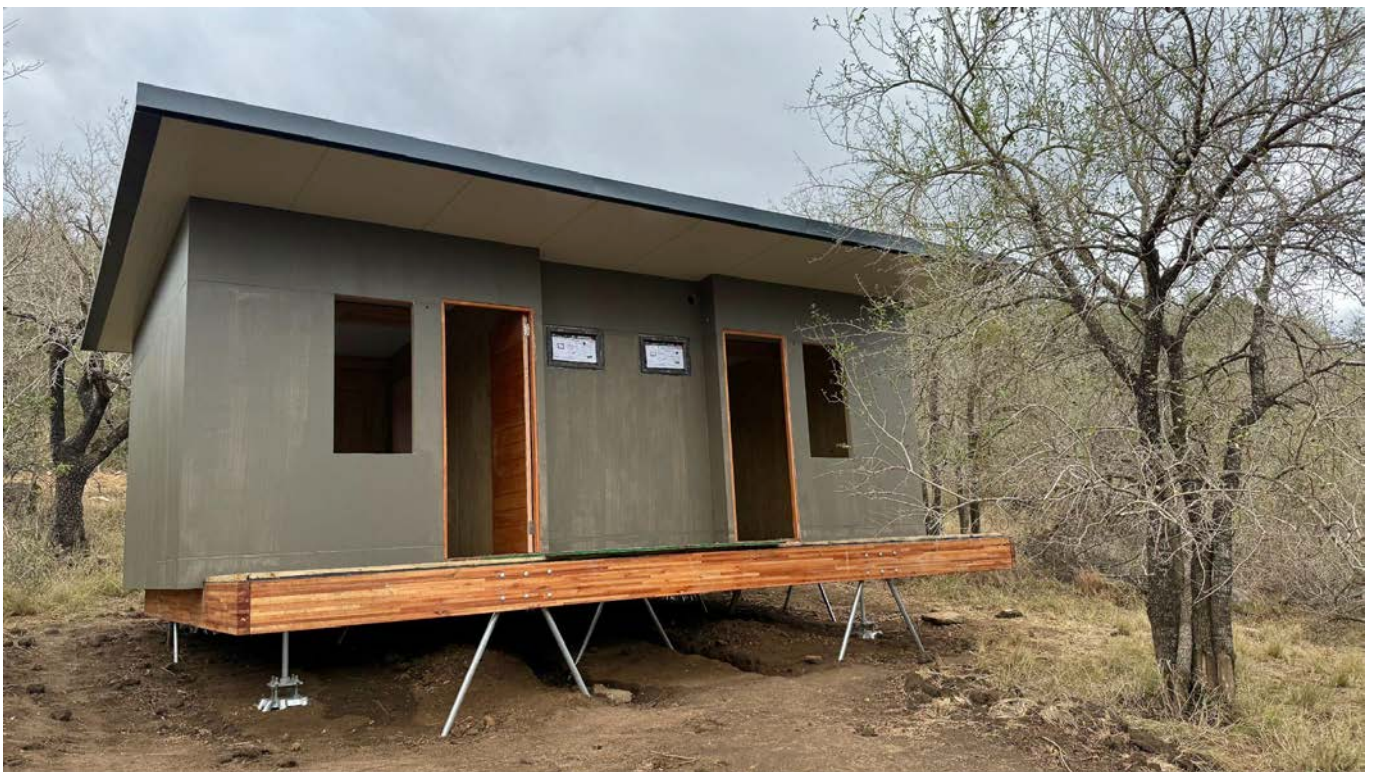
A semi-completed unit. It still needs another coat of paint, the deck and stairs.
